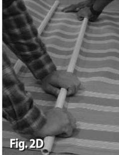
Place the *Bottom Cross Member* (aluminum) underneath the canopy, centering it on the two marks. Position the *Bottom Cross Member* so the punched square holes at the ends are facing downward. Holding the *Bottom Cross Member* in this position, reassemble the *Fabric Clamp* by snapping the *Fabric Clamp* in place at both ends and pressing down, working toward the center (Fig. 2D).
