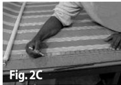
From the back end of the canopy, measure the same distance that was taken off the track length. Make a mark at this distance on both outside edges of the fabric (Fig. 2C).
