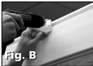
**5** Insert the provided #8 1-1/4" pan head screw into the hole that was drilled in step 4, and secure it into place.
