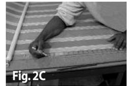
From the back end of the canopy, measure the same distance that was taken off the track length. Make a mark at this distance on both outside edges of the fabric (Fig. 2C).
