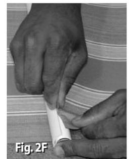
Measure the canopies to ensure the desired length is correct before trimming off excess canopy material. Remove the canopies and place on a flat, clean surface. To remove the excess canopy material, use the edge of the *Fabric Clamp* as a guide when cutting with a sharp utility knife (Fig. 2F).
